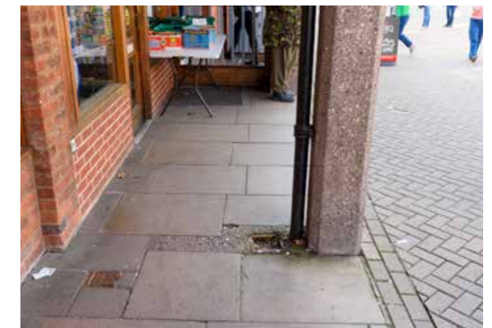
The under-croft area on Bore Street (east)
