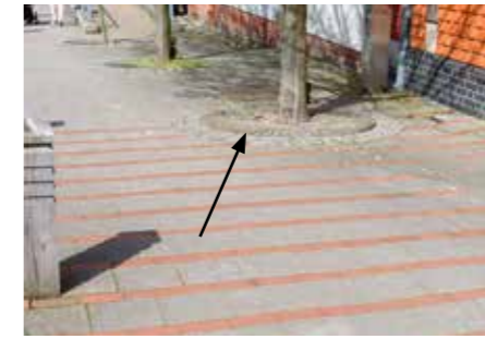
Tree Pit - Circular steel tree grilles, grey concrete block edging
