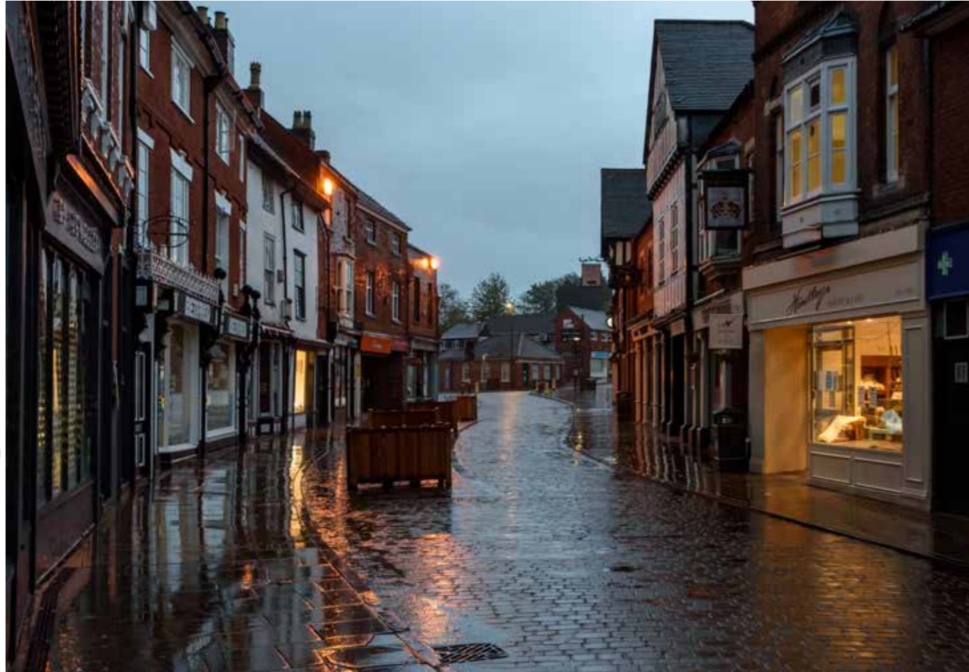
Building mounted light fittings on Tamworth Street
