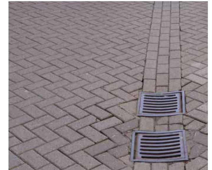
Concrete block paving on Bore Street (east)
