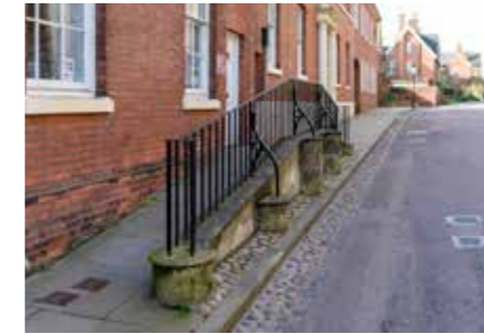
Railings/handrails - Light, black steel
