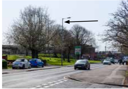
Lighting - 10m highway lighting columns
