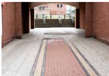
Paving - Red brick blocks set in buff concrete flags with blue and cream coloured brick trims. Blocks of brown concrete paviors set in various coloured brick trims
