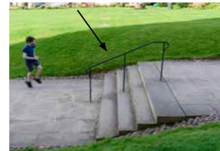
Railings/handrails - Light, black steel
