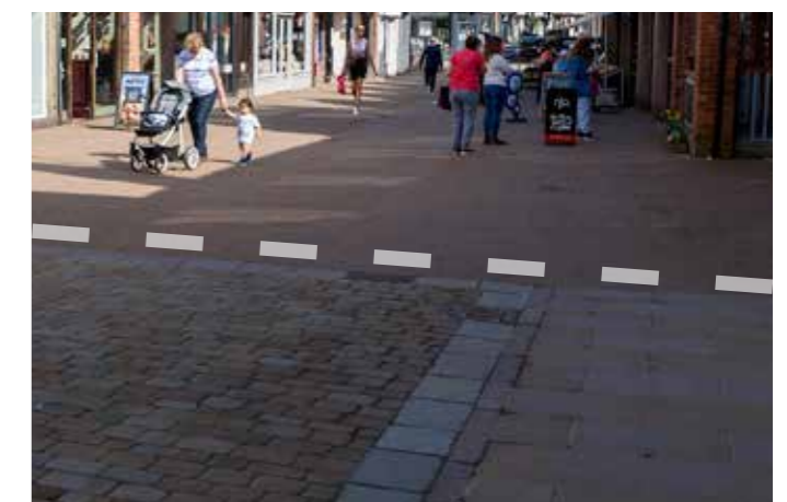
Bore Street East- dashed line indicating the threshold where paving changes from stone to concrete.
