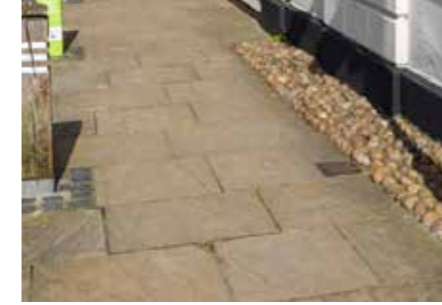
Footpath - Yorkstone to west of junction
