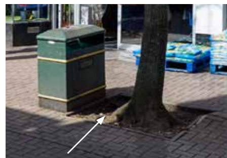
Tree Pit - Square, concrete pin kerbs
