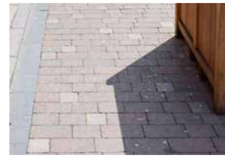
Highway - Multi red concrete paviour
