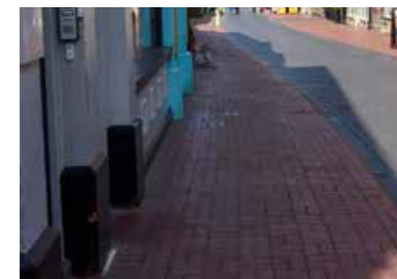
Footpath - Red eng brick (basket weave)
