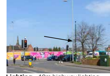
Lighting - 10m highway lighting columns
