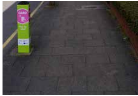
Footpaths - 400 x 400 concrete slabs
