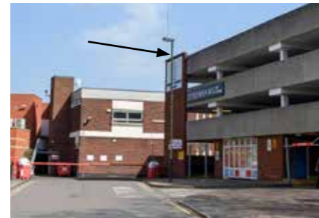
Lighting - Highways lighting columns
