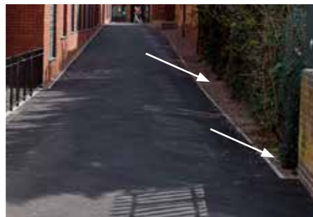
Kerbs - Flush concrete pin kerb and gravel
