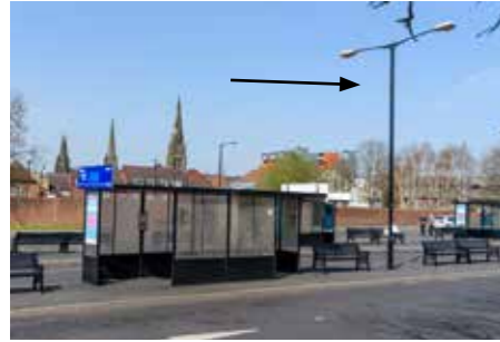
Lighting - 10m highway lighting columns
