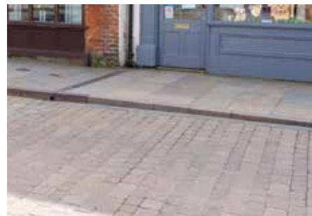
Highway - Concrete tegula paving multi
