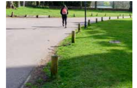
Bollards - Round timber vehicular deterrent
